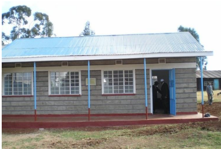
New Ngenia classroom, Outside
