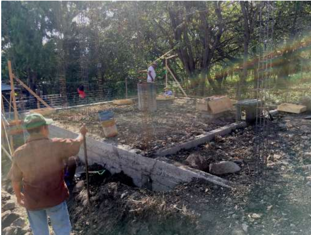
Starting with the foundation
