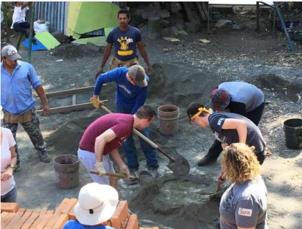
Oregon students mixing cement for building brick walls
