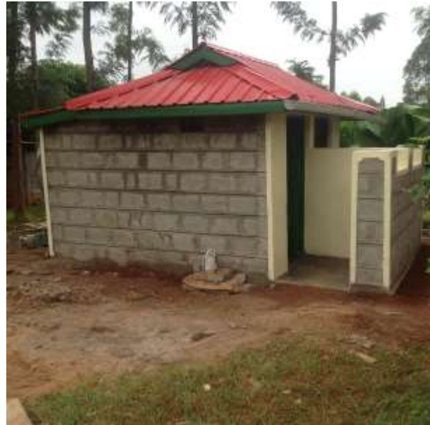
New latrines for another ODFL project completed by same NGO partner, Kiini Sustainable Initiative
